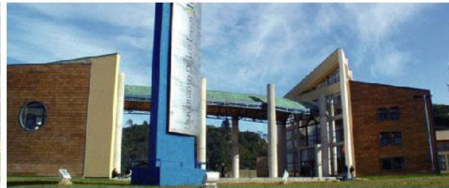
CAMPUS PUERTO MONTT
